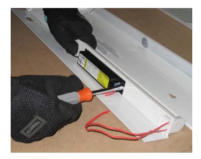
WIRE THE LINE CORD HOT (BLACK) TO BOTH WIRES FROM THE SOCKET (blue in picture). WIRE THE LINE NEUTRAL (WHITE) TO THE OPPOSITE END SOCKET'S WIRES (red in picture) CONNECT THE GROUND (GREEN) WIRES AND SECURE ALL CONNECTIONS WITH WIRE NUTS.
